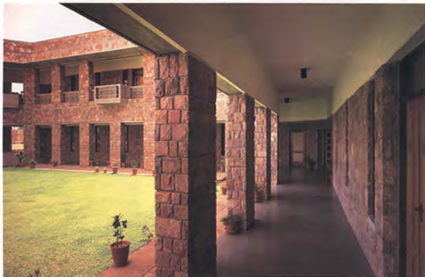
Slender exposed concrete elements are used as a counterpoint against the rugged and vibrant character of stone masonry.
