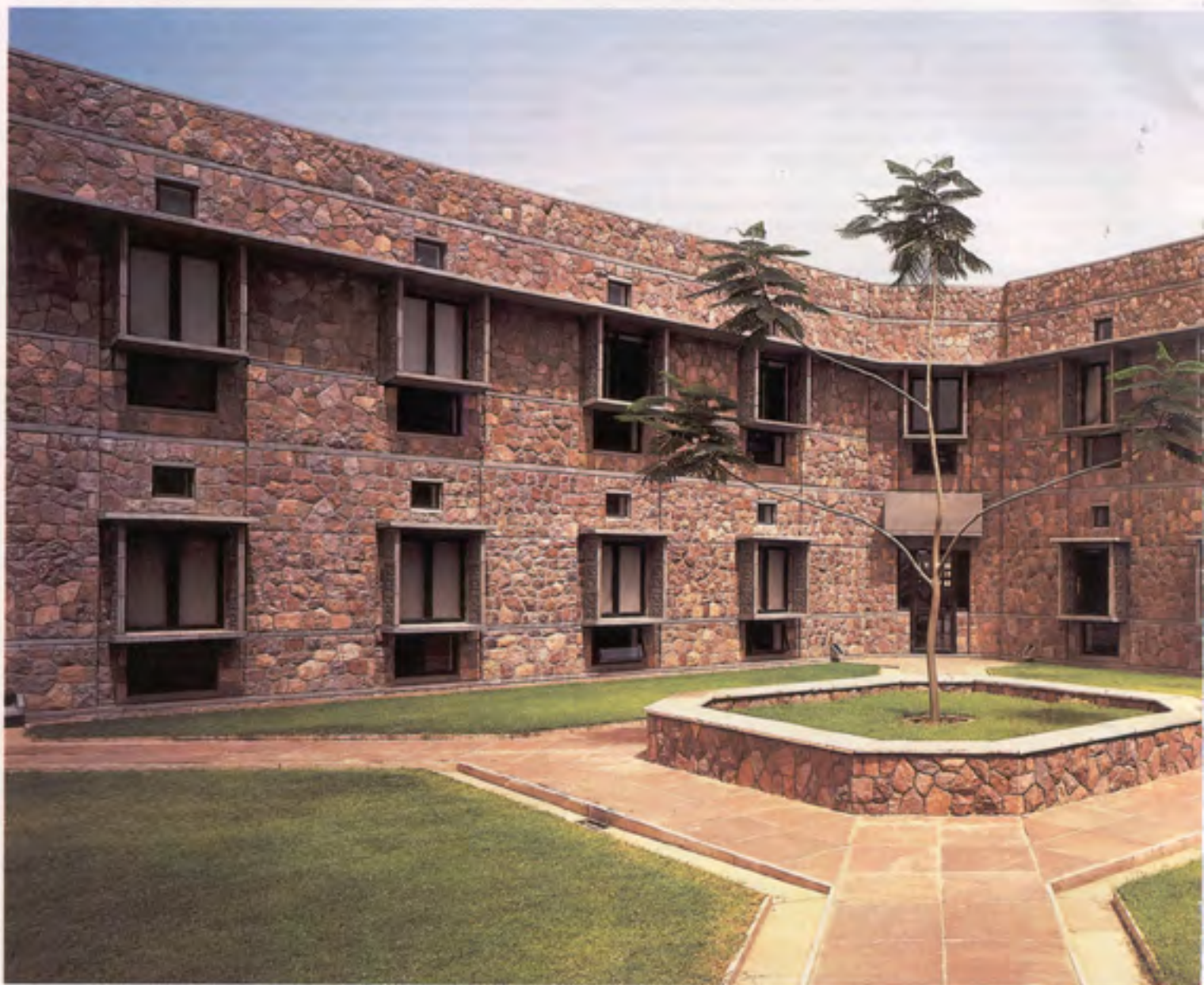
The faculty court — desperately waiting for the tree to give shade and fill out the volume of the court.
