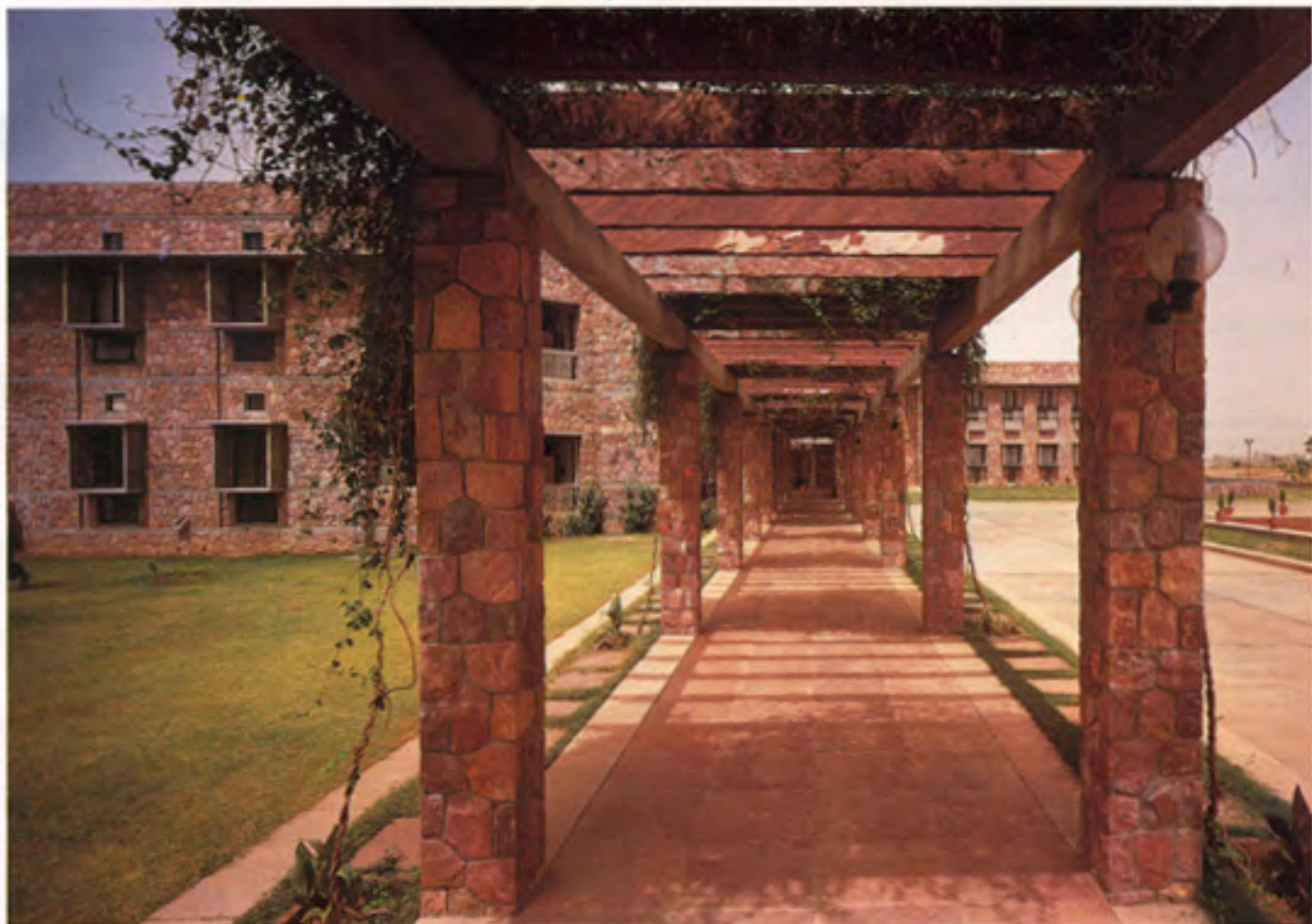
A shaded pergola walk made of stone joists connects the campus gate to the main entrance.
