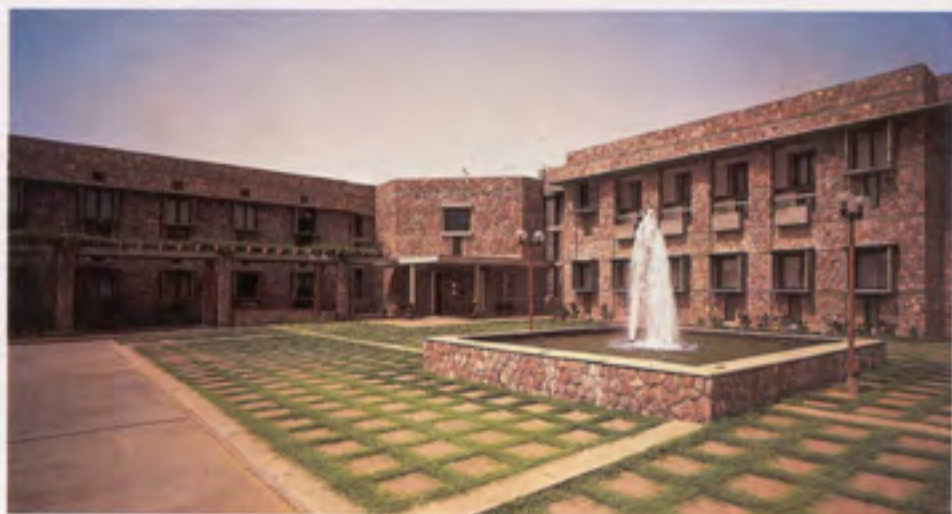
Horizontal bands of concrete give a vertical scale to the buildings while stabilizing the masonry.
