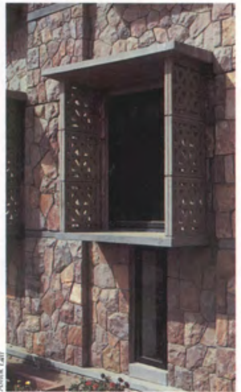
Custom-designed precast concrete jalis are held between precast RC chajjas and sills.
